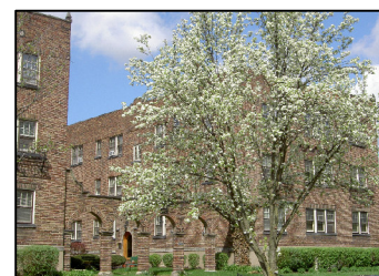
Admiral Apartments Clifton Gaslight Area
